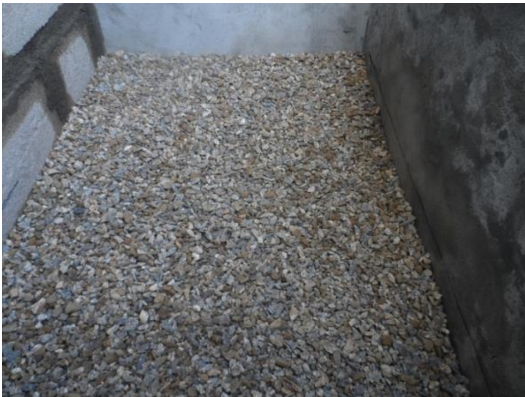
Picture 5: Set-up of the upper layer of the drainage layer, i.e. 10 cm of gravel, Liberia.
