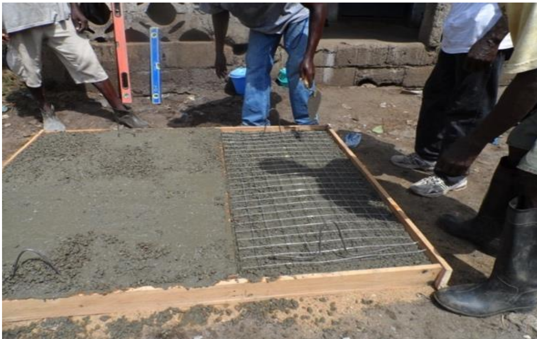
Picture 3: Pouring of a cover slab, Liberia.
