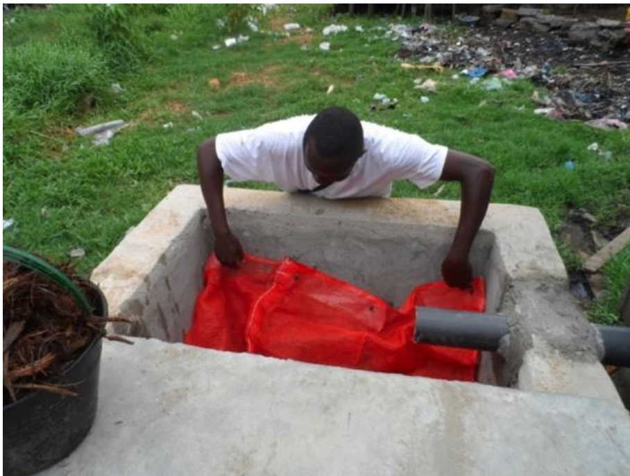
Picture 7: Positioning of onion bags above the drainage layer, Liberia.
