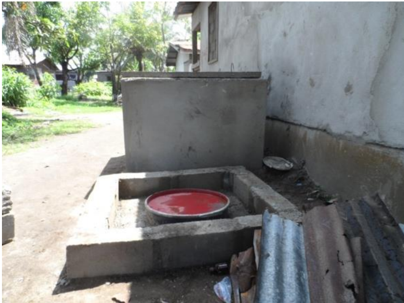
Picture 9: An effluent collector constructed with a plastic drum in Liberia. Protection walls have been raised around the drum to protect it against flooding.
