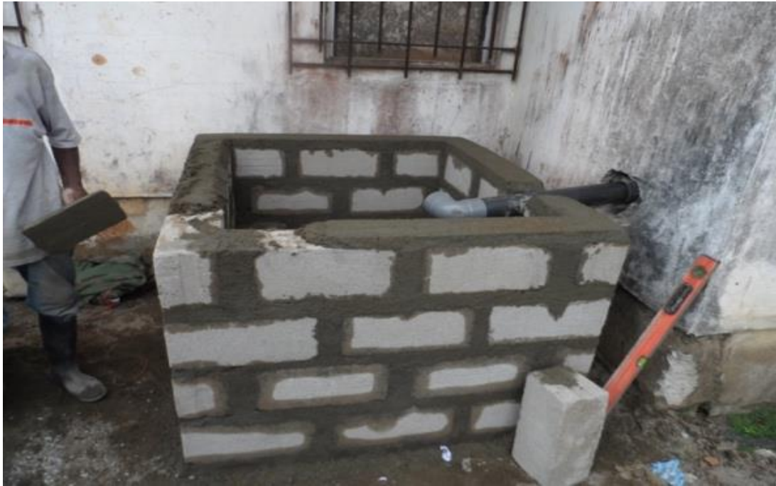
Picture 2: Construction of an above ground biodigester.
