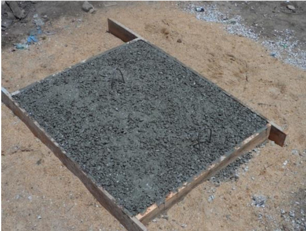
Picture 6: Precast reinforced porous slab, Liberia.
